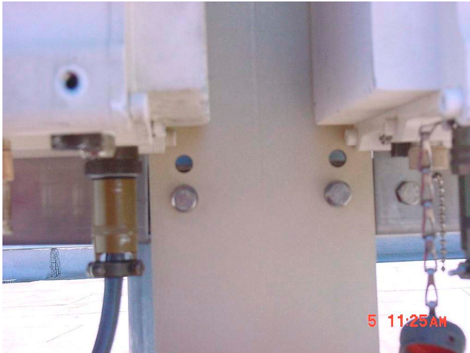
Figure B-19. Position Brackets against Center Bracket.
