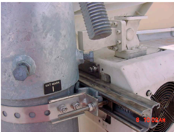
Figure B-4. Installing the Pole Bracket
