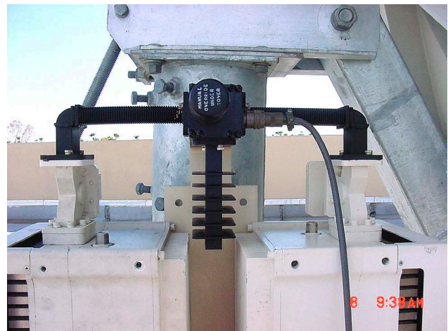
Figure C-19. Installation of the Waveguide Switch.
