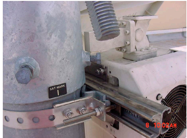
Figure C-4. Installing the Pole Bracket
