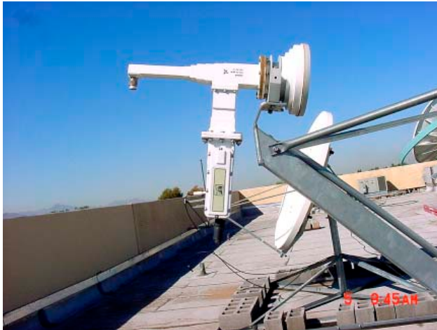
Figure 8-5. Installation of Single-Thread LNA
