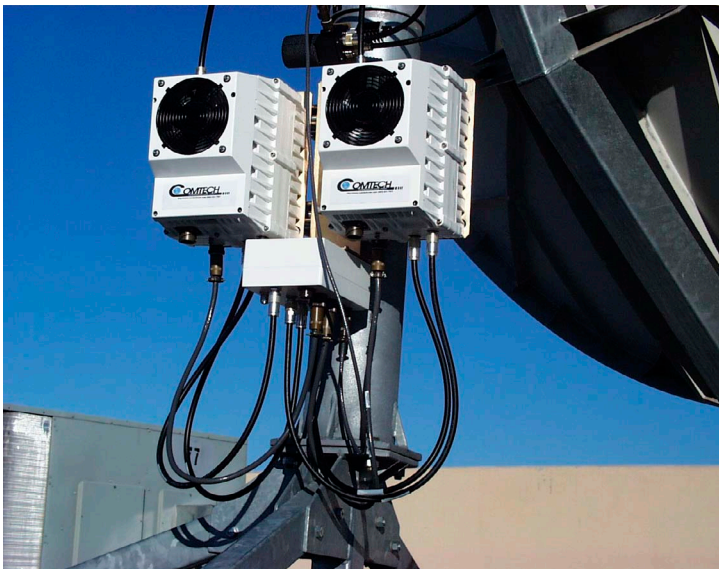
Figure A-23. Cable the Redundant Configuration
