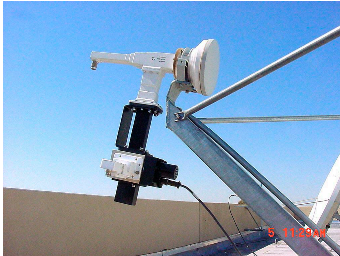
Figure 8-6. Installation of the Redundant LNA Assembly.
