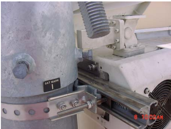
Figure B-4. Installing the Pole Bracket
