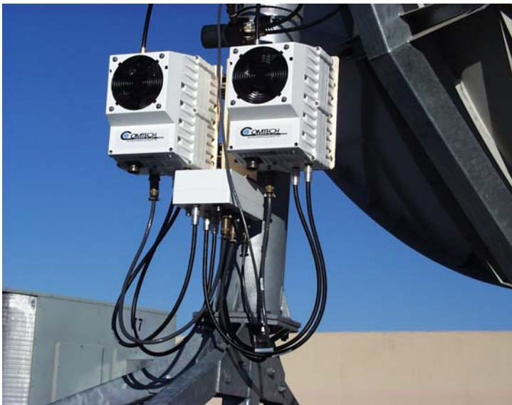
Figure A-23. Cable the Redundant Configuration
