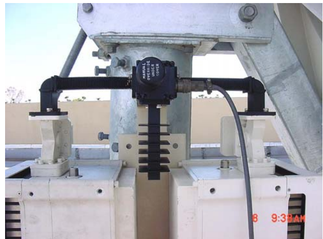
Figure C-19. Installation of the Waveguide Switch.
