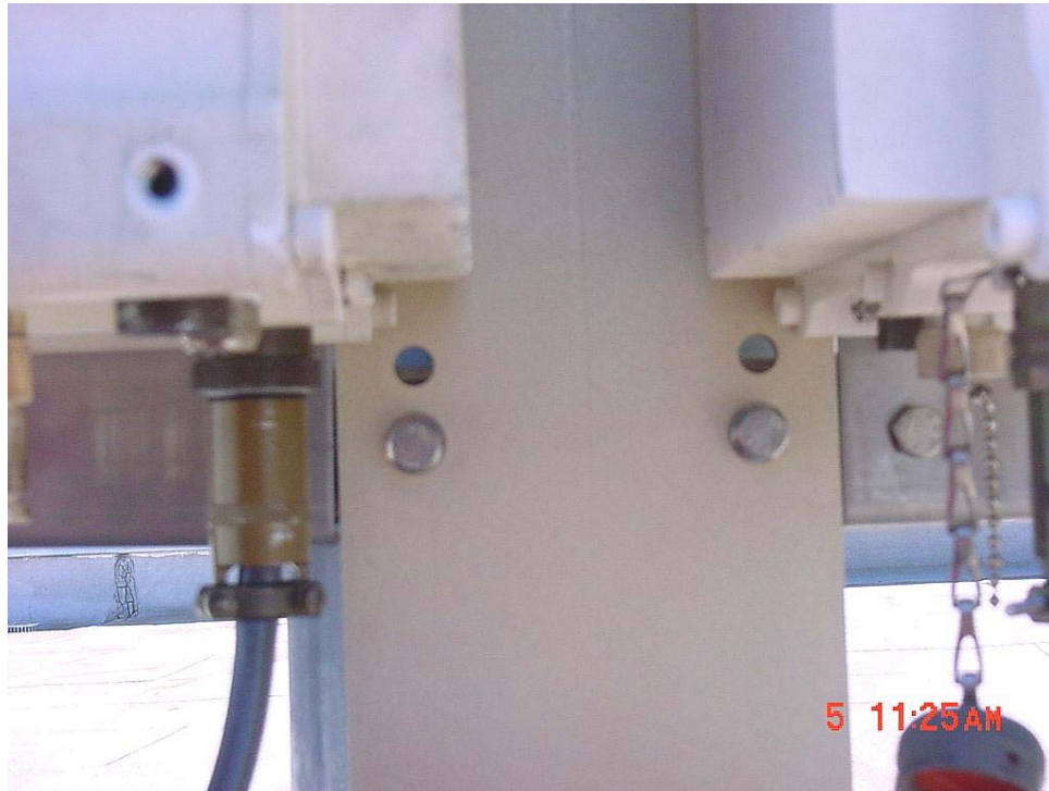
Figure B-19. Position Brackets against Center Bracket.
