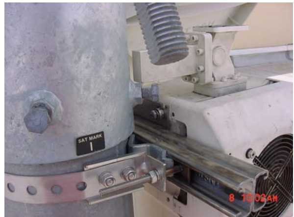
Figure C-4. Installing the Pole Bracket
