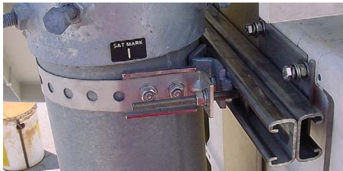
Figure C-16. Pipe Blocks
