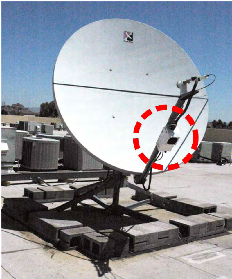
Figure 2-11. SSPA Spar Mount Installation Example
